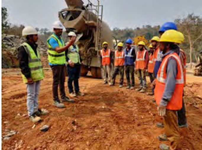
Safety on Concreting Work
