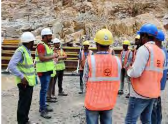
Safety on Concreting Work
