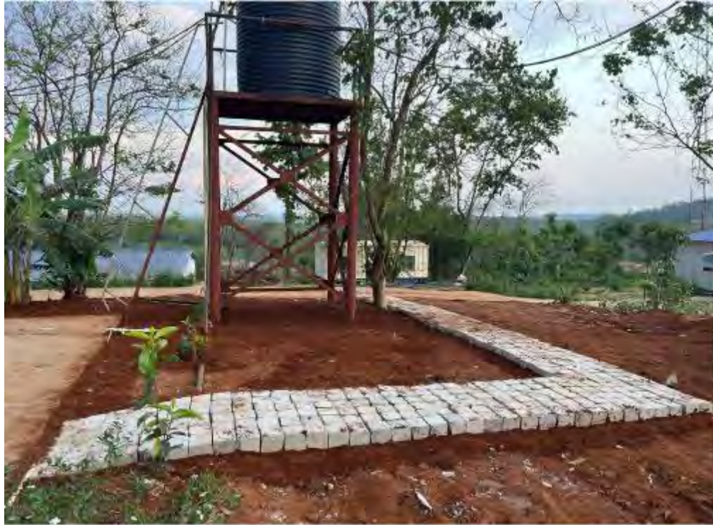
Concrete waste cube reusing for infra work.
